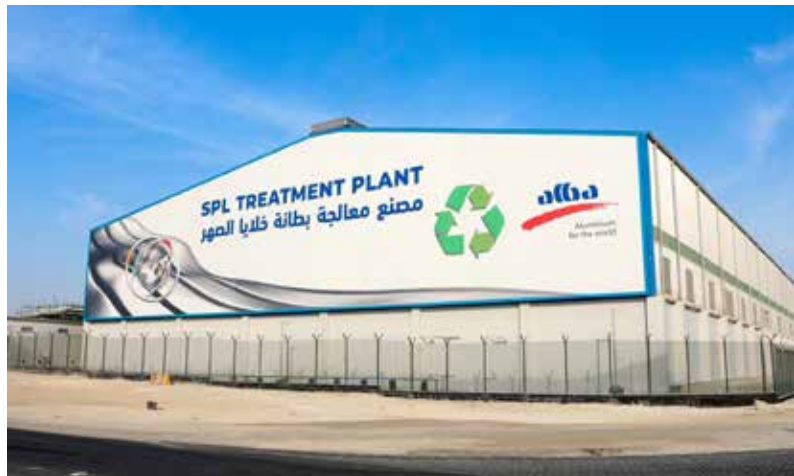
Alba's US$37.5 million SPL Treatment Plant Setting sets a benchmark in sustainability © Alba
