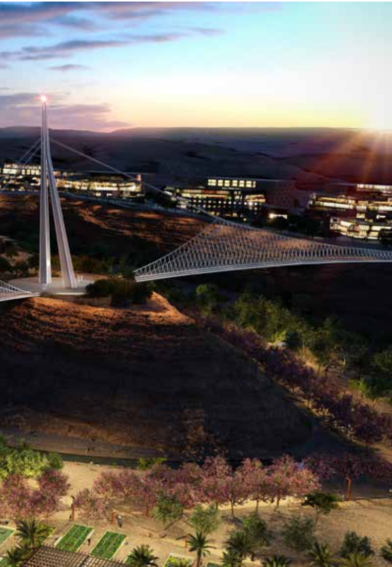
A new landmark in Riyadh: the Lighthouse Bridge is a double cable-stay suspension structure with one central pylon taking the full load of the two 200m long spans. © AS+P Albert Speer + Partner GmbH / visualization: V1
