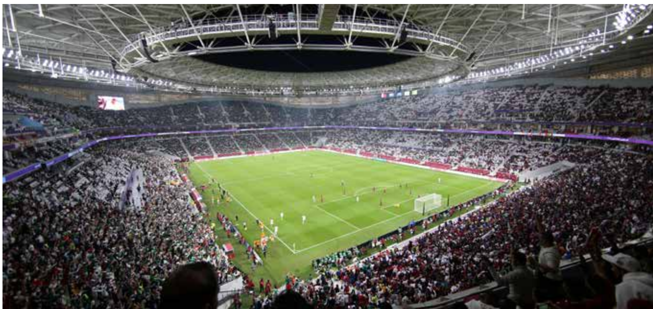
Inside view of the Al Thumama Stadium. Wilo supplied solutions for water supply as well as pressure boosting © Wilo
