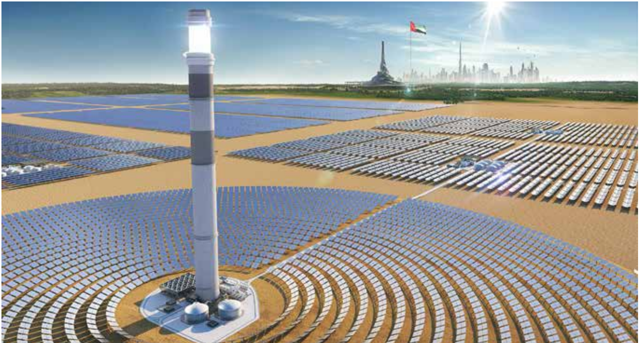
Legend: In a solar tower power plant, such as the one used in the Noor Energy 1 project, the sunlight is reflected from several hundred mirrors to a central tower. © Noor Energy 1
