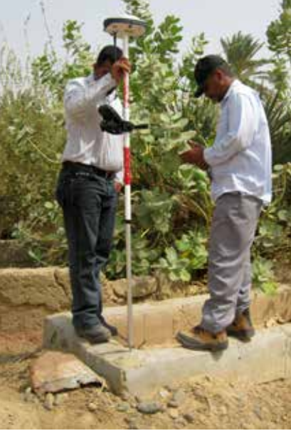
Topographic survey works at Zahban dam
