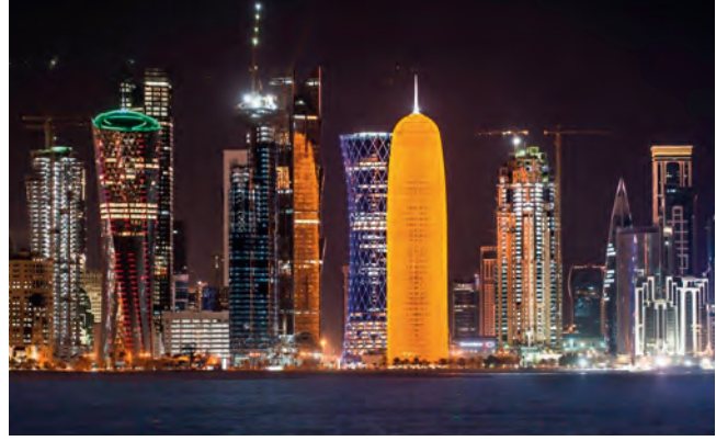
instalight 1050 – Façade Spot – Standing Out: 3.362 LED façade spots with a total power consumption of 180 kW illuminate the tower with sequences in gold and platinum/silver. Photo: Stefan Tornau, Qatar
