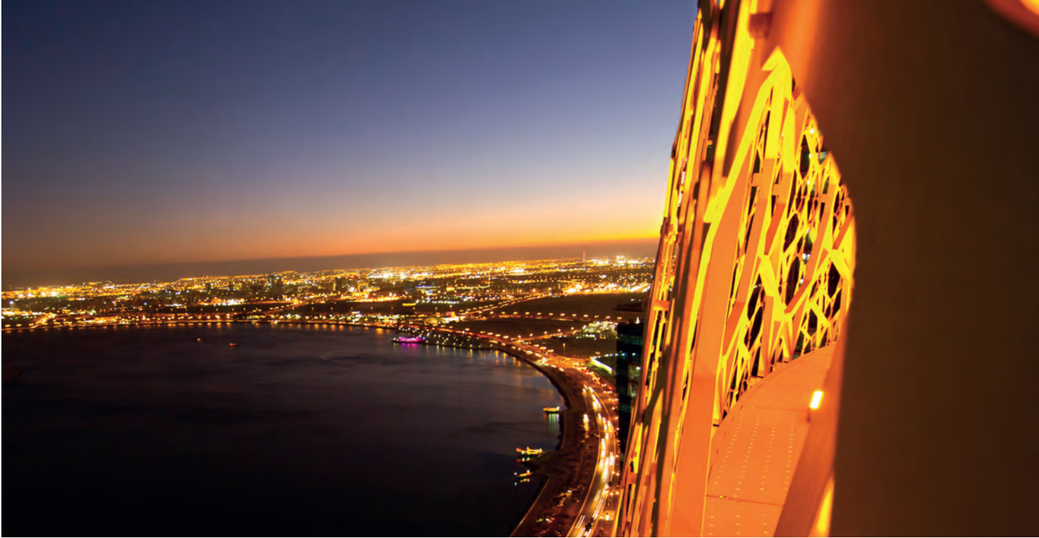
instalight 1050 – Façade Spot – The golden LED light is covering the mystic ornaments of Burj Doha, providing changing reflections, shadows and brilliance. Photo: Stefan Tornau, Qatar
