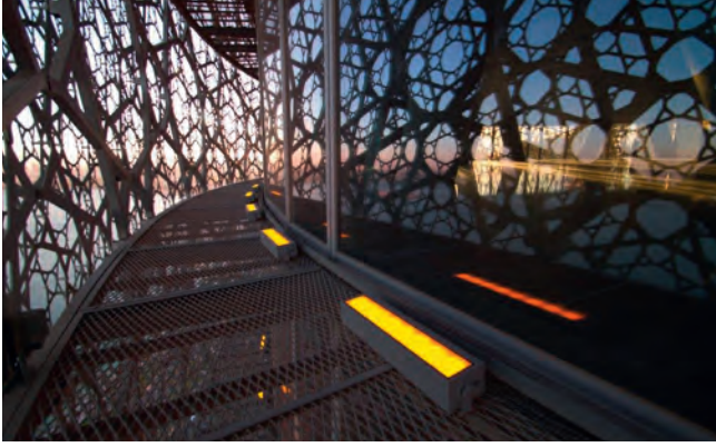
instalight Control – 10.086 channels control the luminaires with integrated temperature management. Photo: Stefan Tornau, Qatar
