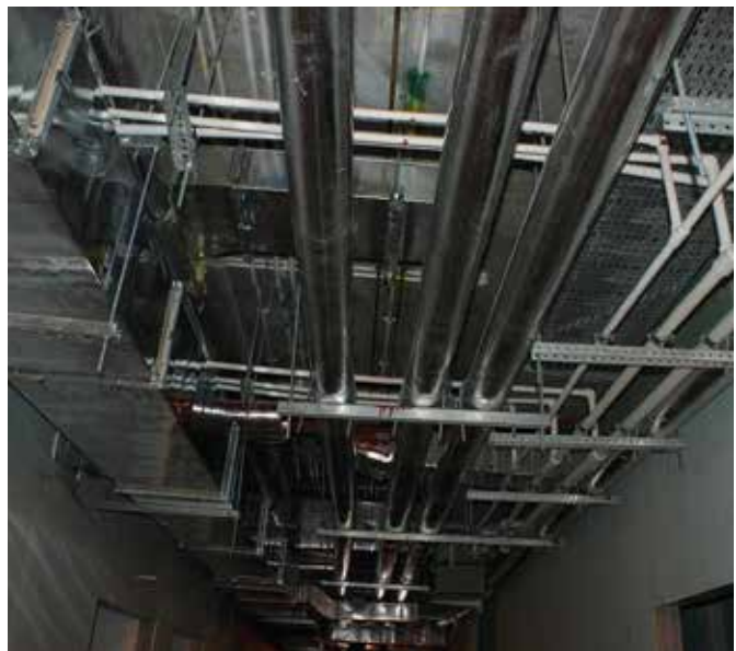
3 | Electro- mechanical constructions in Al Najaf Teaching Hospital
